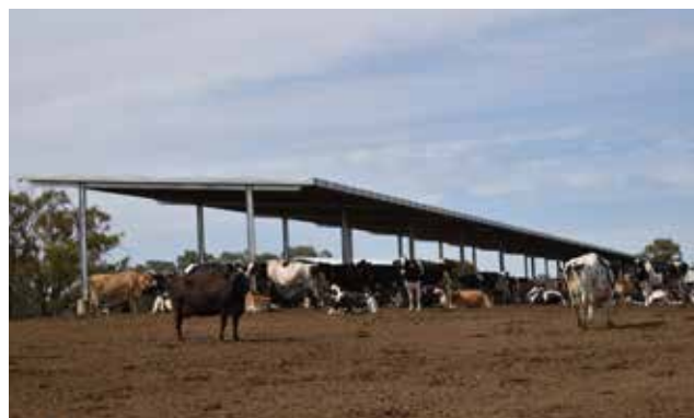
Figure 26. Centralised shade shelters at a dairy dry lot with a north-south orientation
