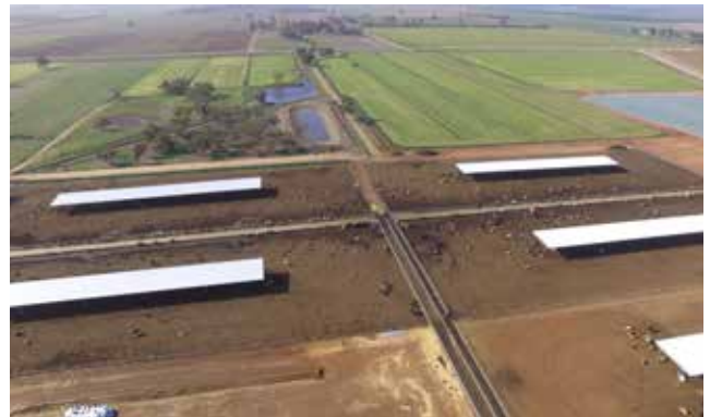
Figure 29. Aerial image of a well-designed dairy dry lot with north-south shade structures and central feeding table
