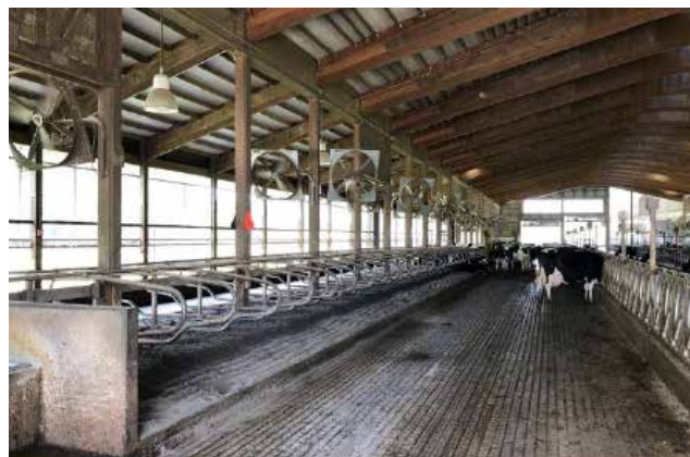
Figure 77. A naturally ventilated freestall with two-row head-to-head stalls
