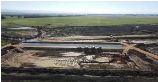
Figure 9. Construction of an earthen feedpad and ponds – long view
