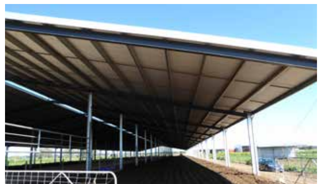
Concrete roofed feedpad with dry scrape feed alleys
