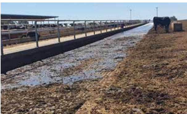
Flood washing of concrete cow feeding alleyways
