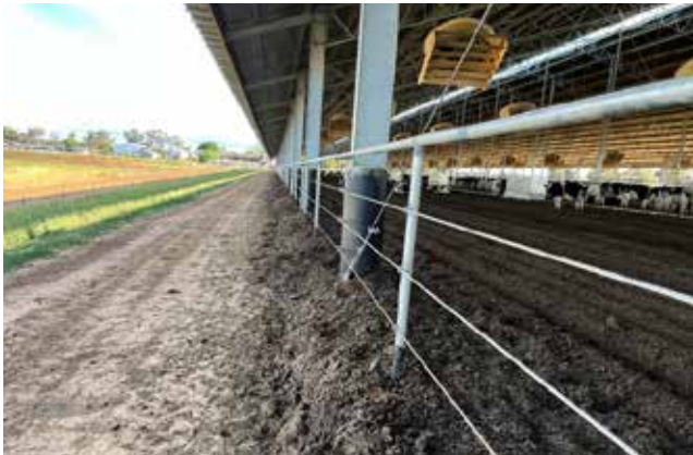
Figure 41. Eave overhangs can help minimise the amount of wind, precipitation, and sunlight entering the housed facility
