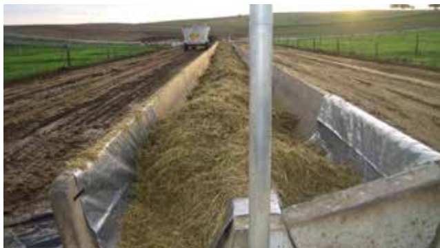
Formed earthen feedpad with concrete troughs
