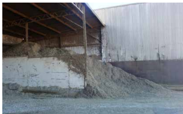
Figure 90. Design individual bays to cater for typical delivery truck volumes – store feed undercover
