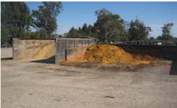
Concrete bunkers for storing by-products
