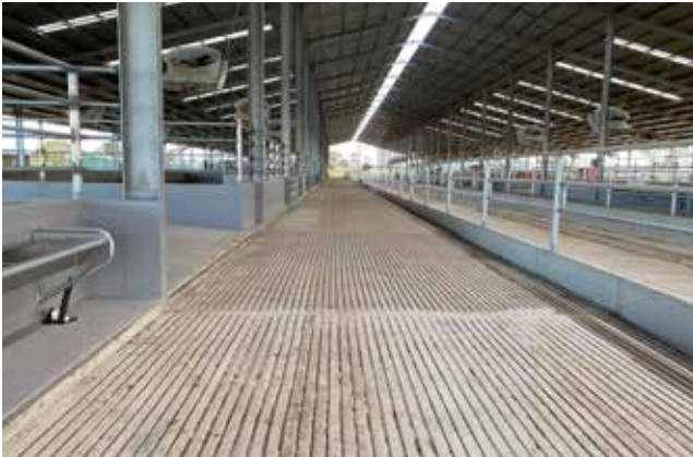
Figure 69. Concrete grooves on flooring
