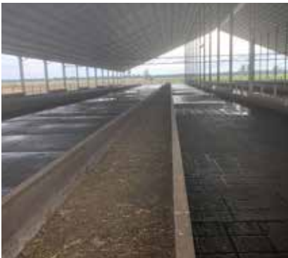
Concrete roofed feedpad with multiple rows of feed troughs
