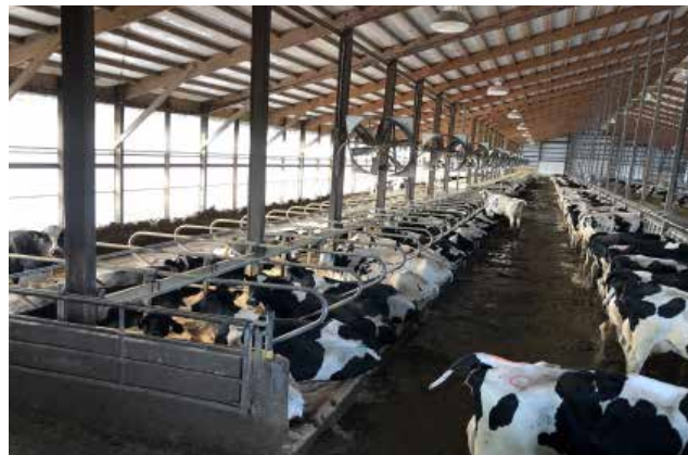
Figure 55. Two-row tail to tail freestall pen
