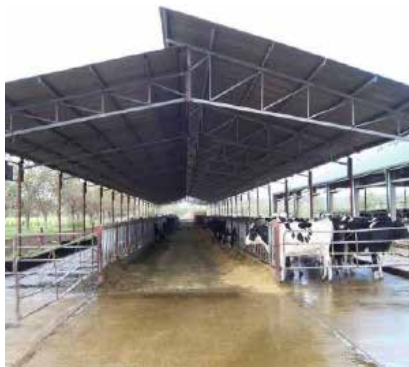
Concreted overlapping roofed feedpad
