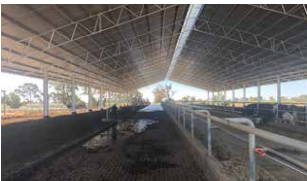
Concrete roofed feedpad with extended eaves for cattle loafing
