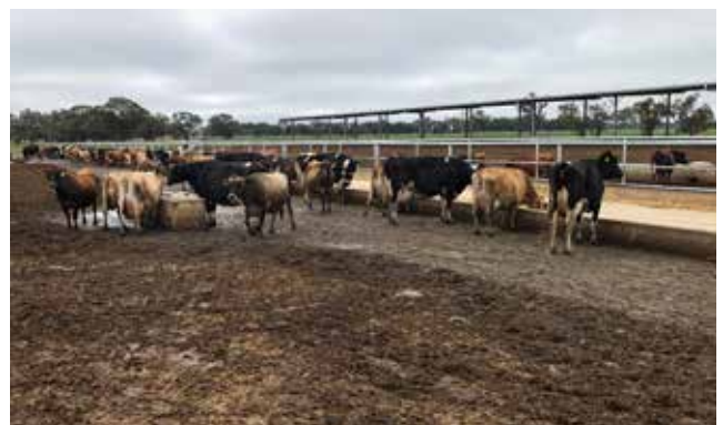
Figure 30. A leaking trough will cause drainage problems on the earthen dry lot pen
