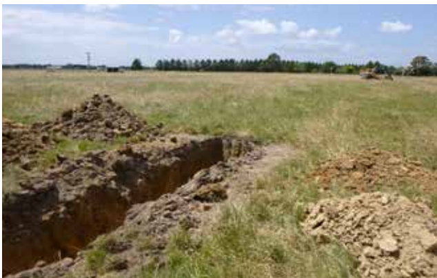
Figure 4. Layers of soil extracted from investigation sites using an excavator
