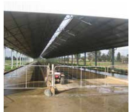
Fully concreted feedpad with nib wall, central feed alley, solid roof and flood wash system
