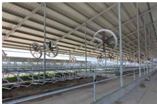
Figure 78. Fans over freestalls and the feeding table
