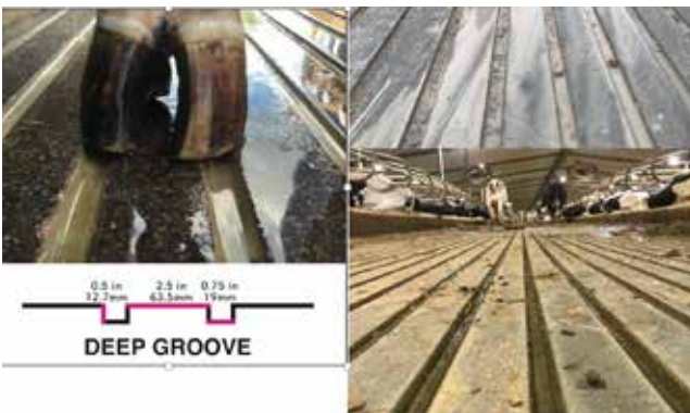
Figure 70. A deep groove pattern provides the best traction for cows
