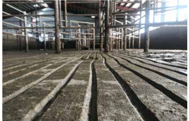
Figure 72. V-shaped groove patterns should be avoided as they result in more slips and an increase in lameness
