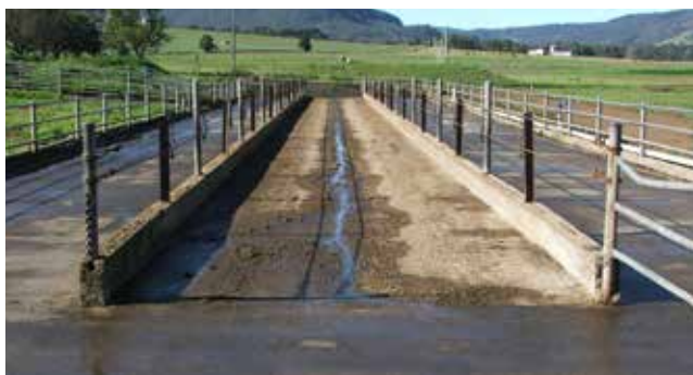
Concrete feedpad with separate drive and feed alleys
