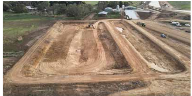
Figure 10. Construction of an earthen feedpad and ponds
