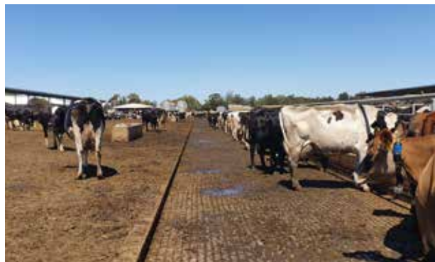
Concrete cow feeding alley ways constructed with a nib wall against the dry lot to prevent the runoff reaching the earthen surface of the pen
