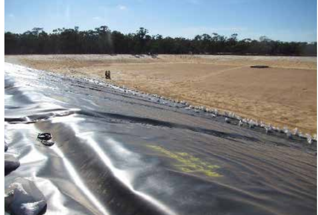
Figure 8. HDPE lining installed for impervious ponds in northern Victoria
