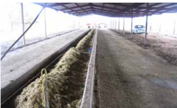
Wider square-profiled trough on earthen pad under solid roof
