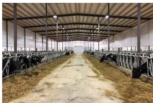
Figure 79. Cross ventilation system with curtain baffles to direct fast-moving air into the resting area
