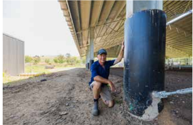
Figure 80. Posts encased in PVC and concrete protect the steel from corrosion
