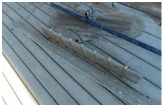
Figure 73. A typical float used to groove wet concrete
