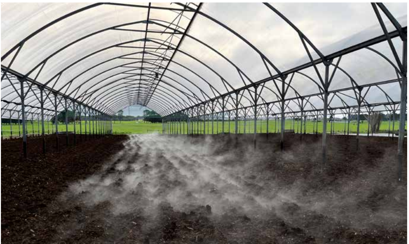
Figure 25. Cattle shelter with a steel frame and flexible clear roof membrane.
