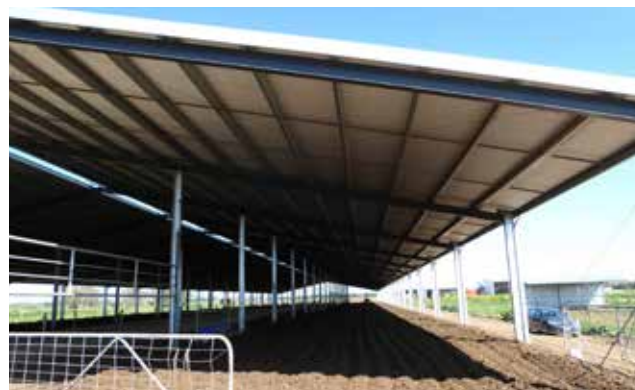
Concrete roofed feedpad with dry scrape feed alley
