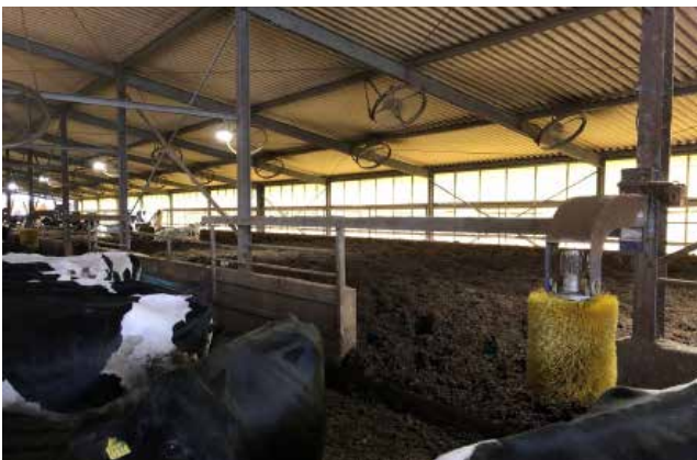
Figure 39. Compost bedded pack – high retaining walls, barriers stop cows climbing over wall if bed is full
